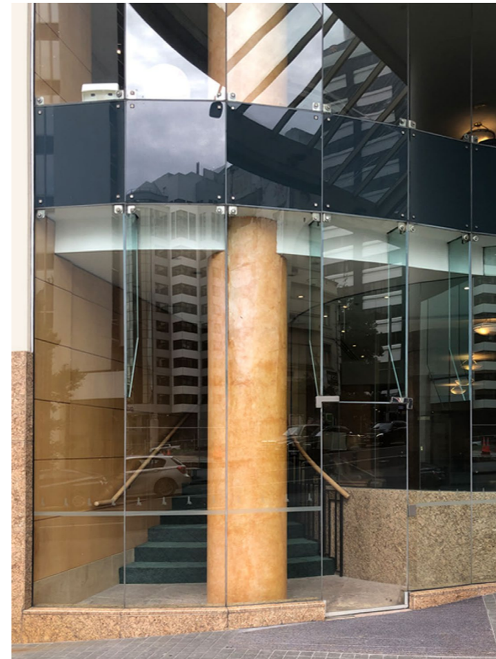
▲ Previous side entrance, view from exterior. Originally a restaurant entrance.
